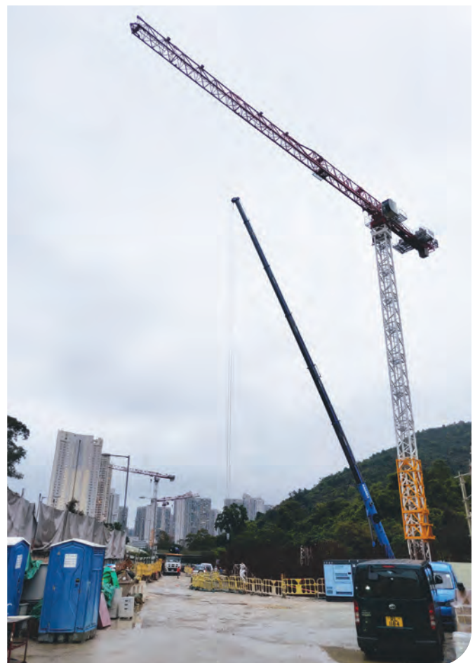
ABOVE: The five tower cranes arrived on site between March and May of 2020, and they are expected to stay until 2022.
