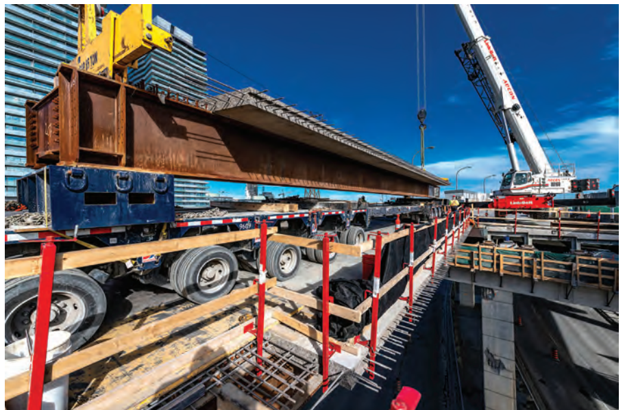
TOP: The Strategic Rehabilitation Plan by the City of Toronto will revitalise the 62-year-old expressway in multiple phases.
