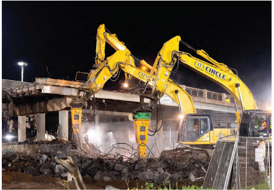
ABOVE AND BELOW LEFT: Indeco HP 5000 and HP 7000 hammers played an important role in the demolition of the Duncan Road bridge and the safety barriers of the pillars.
