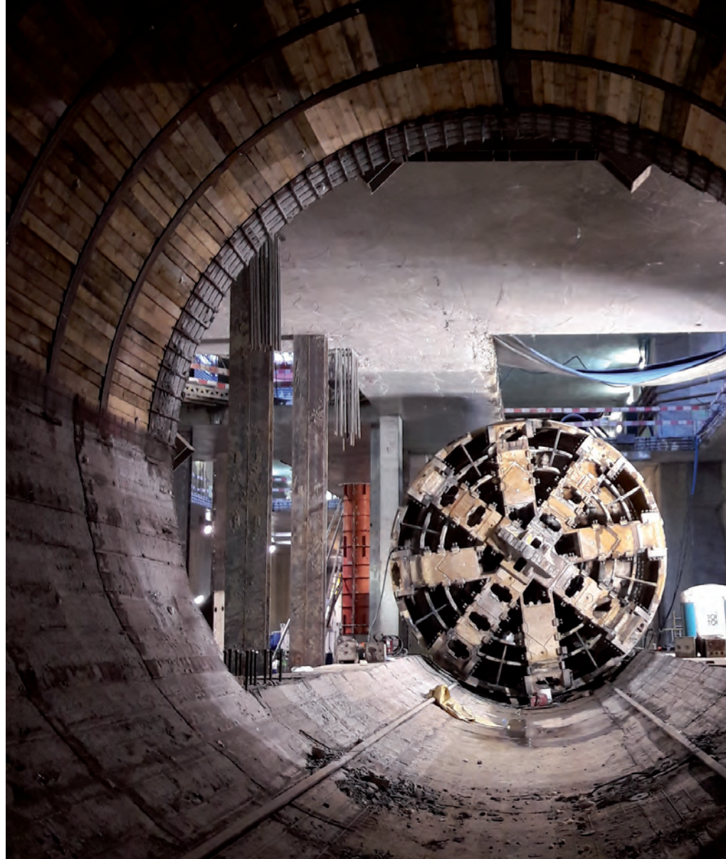
The excavation of the tunnels involved the use of two EPB TBM machines.
