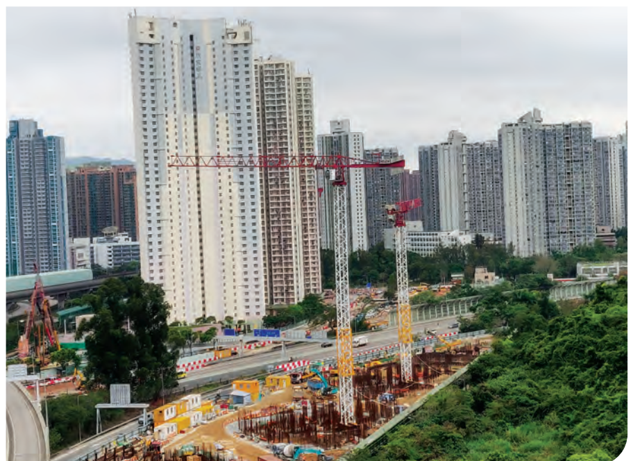
TOP AND ABOVE: The new residential development is being built with the help of Potain tower cranes. Managed by the Hong Kong Housing Department, the project will have five towers ranging from 37 to 40 storeys upon completion.
